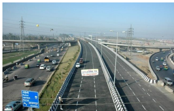
Fig: 3. Completed View of Mukarba Chowk Grade Separator
