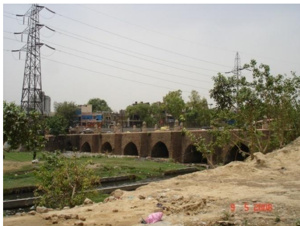
Fig: 20. No Physical Disturbance to Heritage Structure
