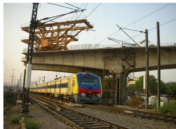
Fig: 19. No Disturbance to Rail Traffic during Precast Segmental Construction
