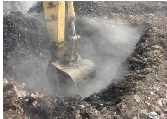
Fig: 11. Excavation in the Landfill Area
