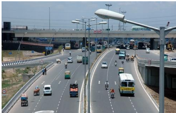
Fig 4: View of Azadpur End
