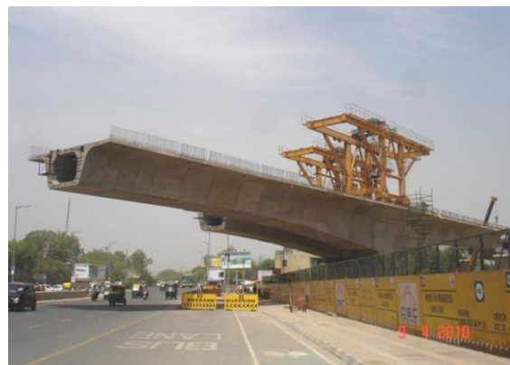
Fig: 18. No Disturbance to Road Traffic during Precast Segmental Construction
